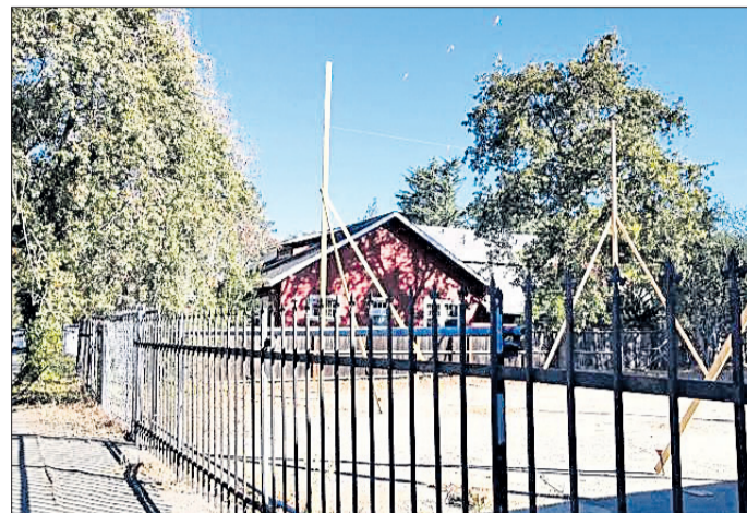
Story poles went up this fall at the site of the proposed Gateway Project on Broadway. The mixed-use development narrowly won approval from the city.
